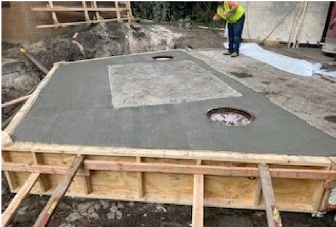
Pictured above: Crews have formed part of one of the large underground concrete structures.
