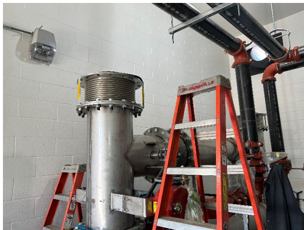
Exhaust Heat Exchanger Piping Installation
