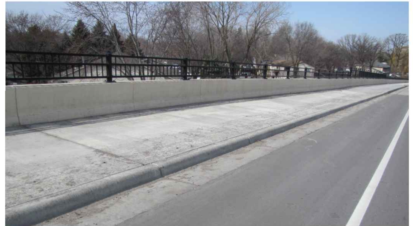
BRIDGE APPROACH TYPE: TRAIL AT BACK OF CURB & GUTTER PROJECT: HANSON BLVD. OVER BNSF RAILWAY CO. LOCATION: COON RAPIDS, MN
