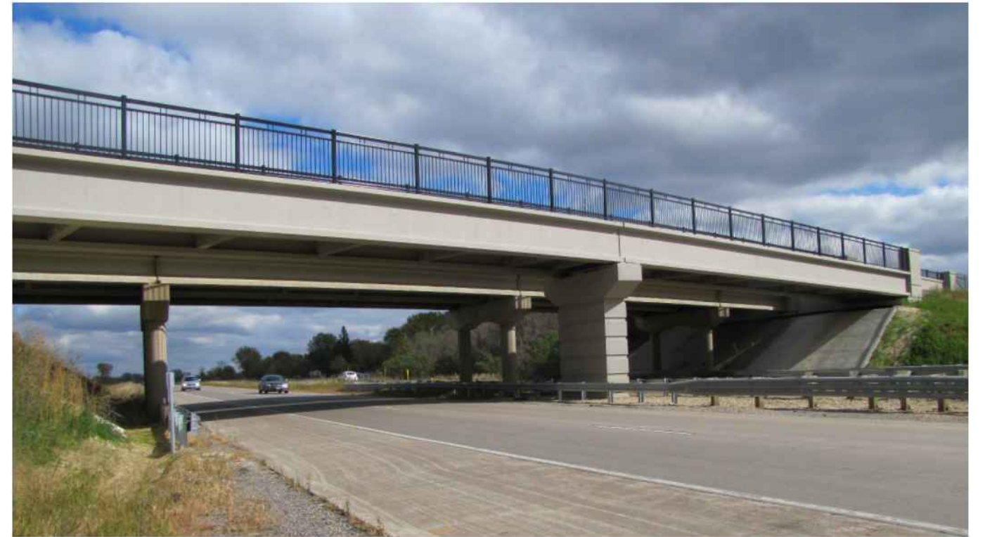
BRIDGE TYPE: PRESTRESSED CONCRETE BEAM W/ THRU GIRDER DECK PROJECT: CSAH 14 TRAIL BRIDGE OVER I-35W LOCATION: LINO LAKES, MN
