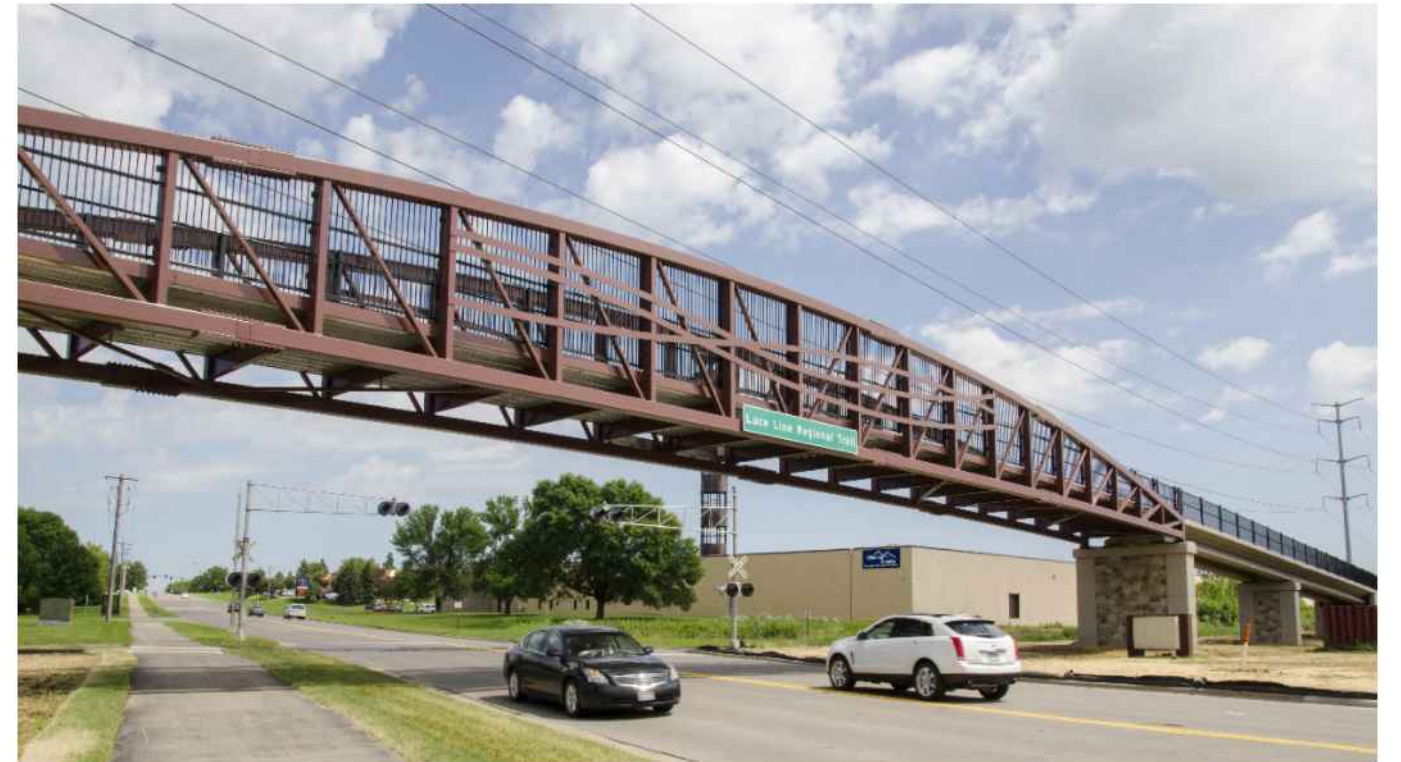
BRIDGE TYPE: PREFABRICATED STEEL TRUSS PROJECT: LUCE LINE REGIONAL TRAIL BRIDGE OVER CSAH 61 LOCATION: PLYMOUTH, MN
