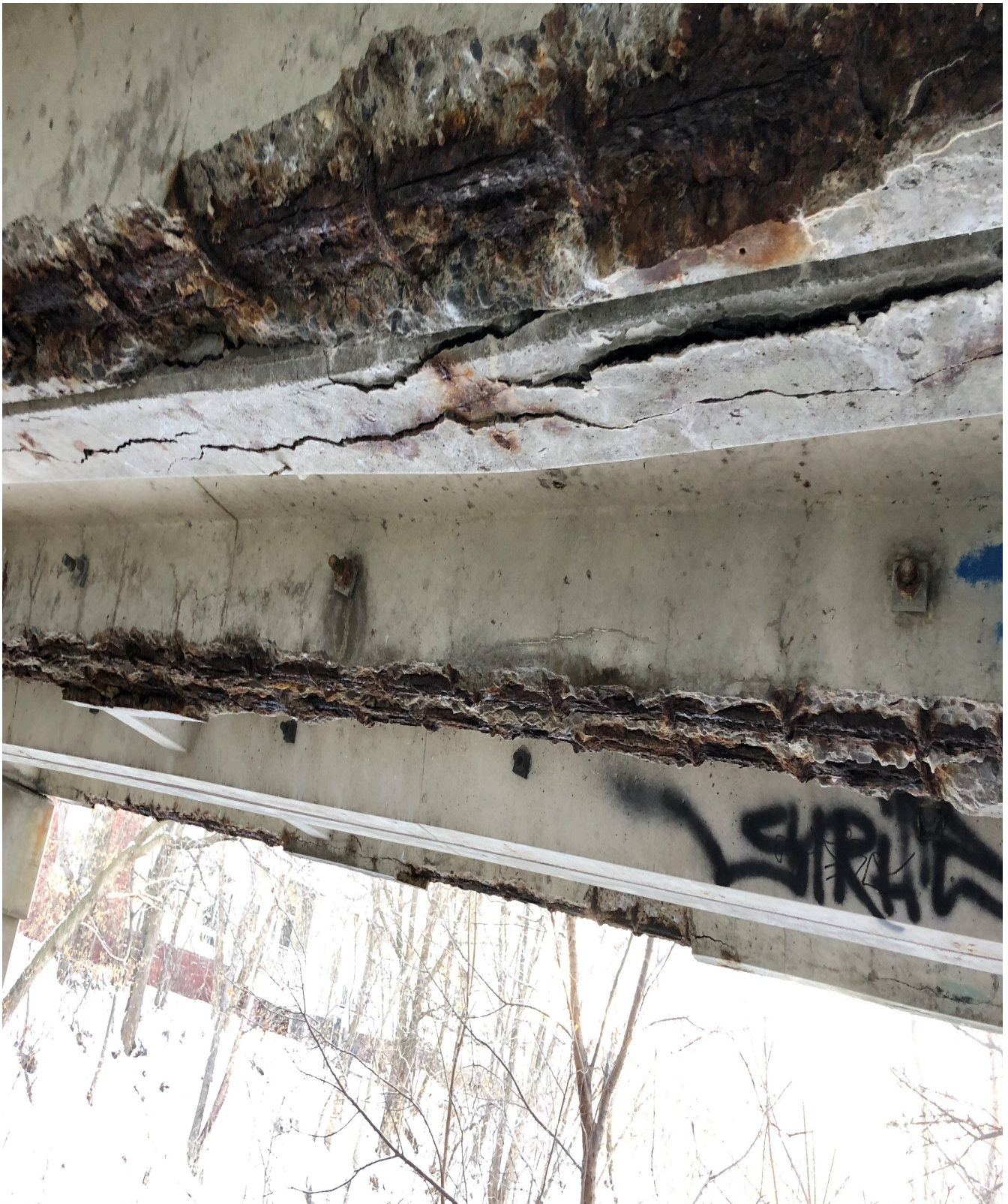
Bridge 4533 beam condition showing section loss
