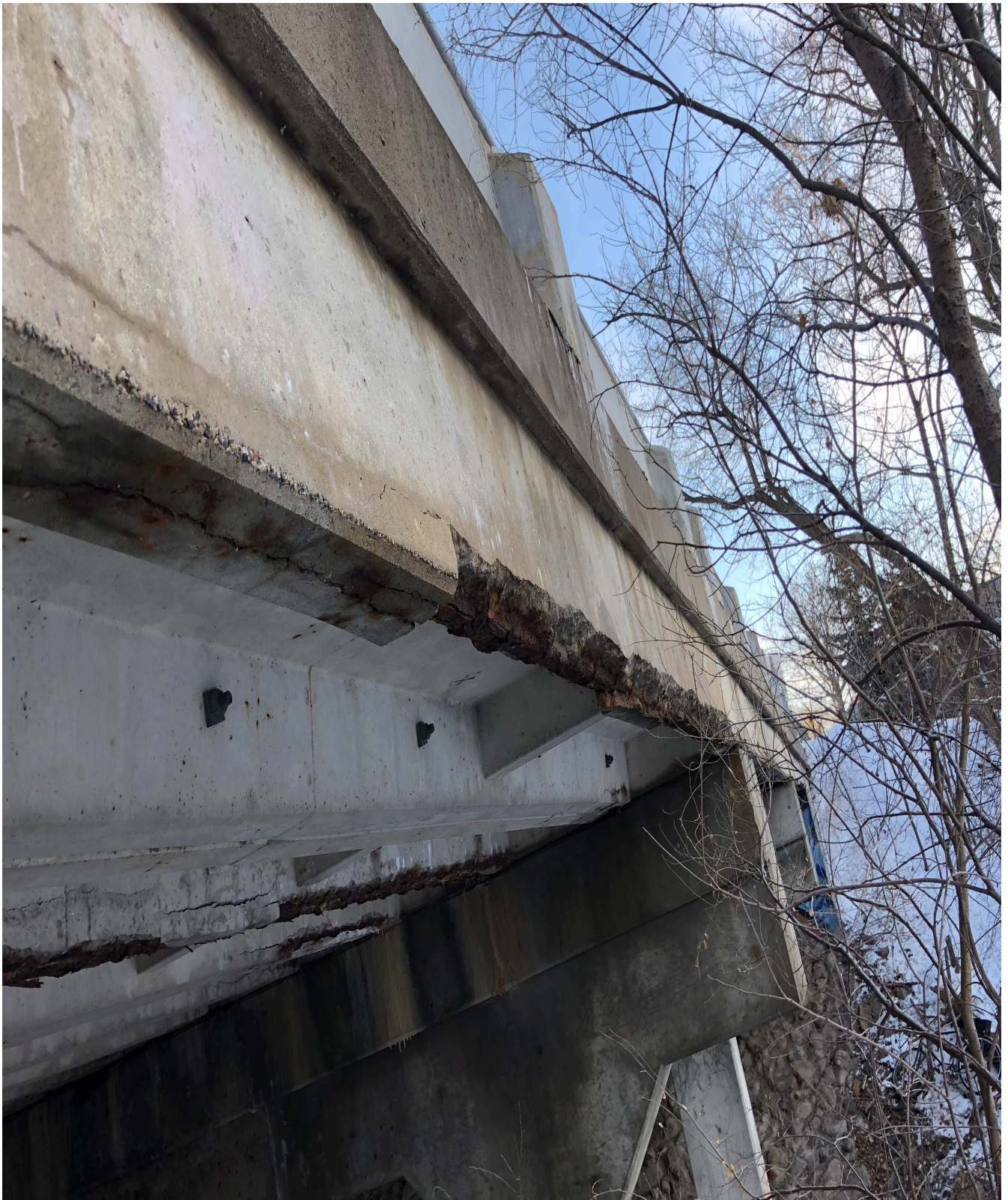
Bridge 4533 exterior beam showing section loss
