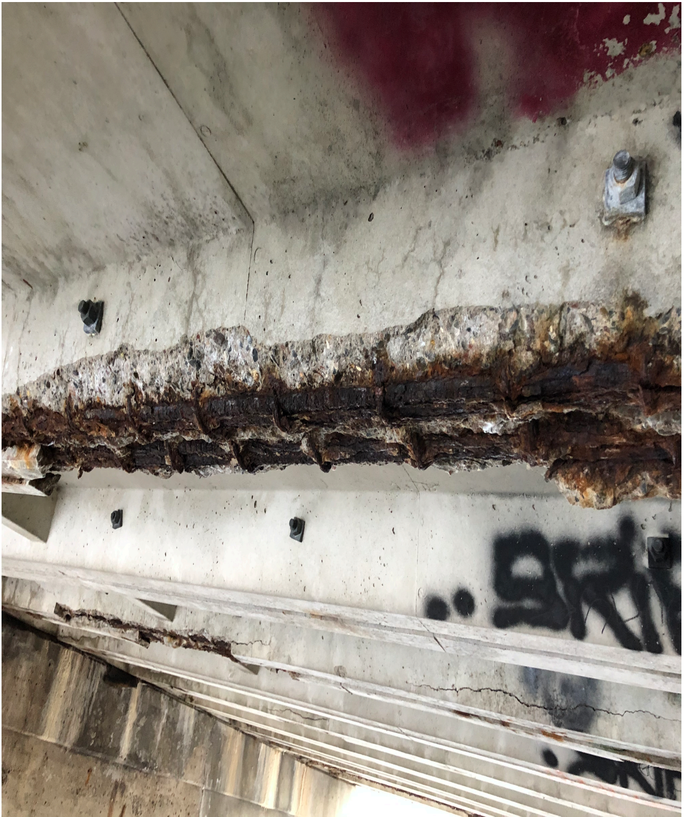
Bridge 4533 beam condition showing section loss
