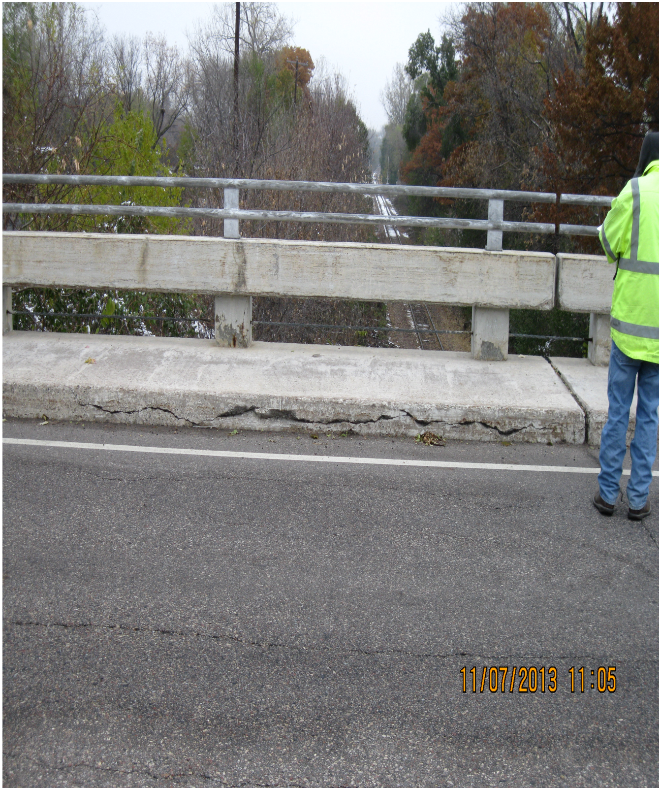
Crack and deterioration of north curb.
