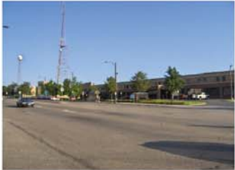
Large radio towers and office space.
