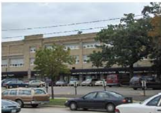
Storefront interests have populated the ground floor of the Griggs building.
