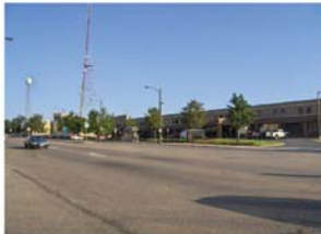
Large radio towers and office space.
