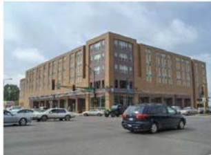
New library: southwest corner of Dale & University.
