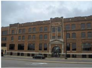
Classic building stock is an asset to the station area.
