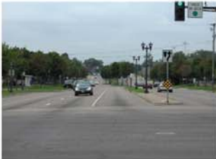
Lexington Parkway adds a 'green' component to the station intersection.
