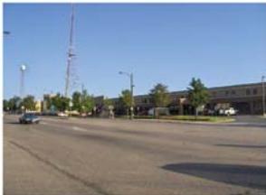
Large radio towers and office space.
