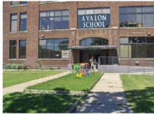
Adjacent uses include this public school.
