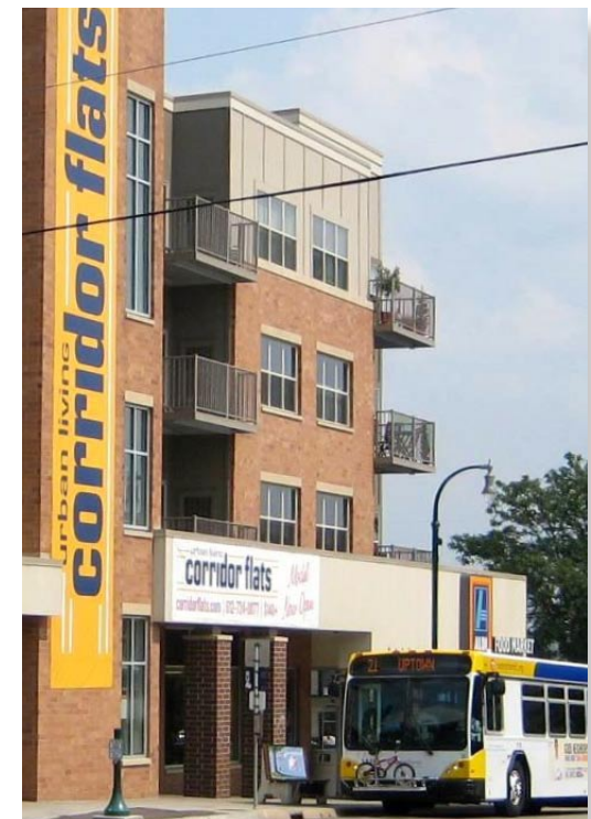
Figure 4-2: Development density impacts the types of efficient transit service available to communities
