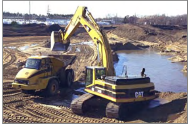
Construction of a stormwater retention pond for park
