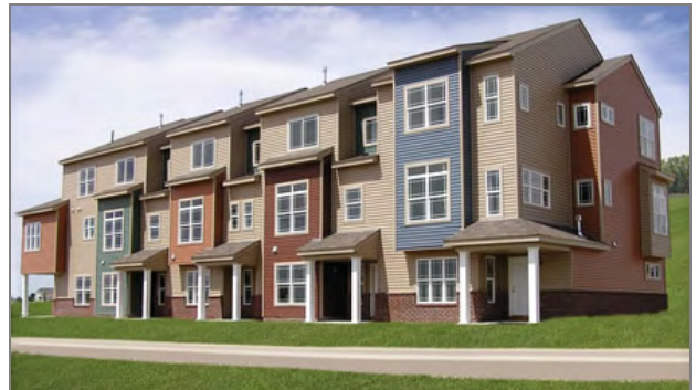
Construction of 103 townhomes, built by D.R. Horton, began in the fall of 2004
