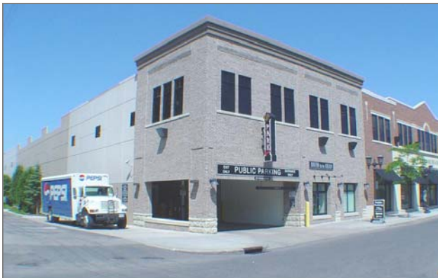
Parking ramp entrance and rear service entry
