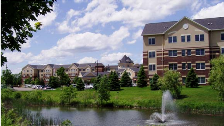
Boutwells Landing in Oak Park Heights: a range of levels of care to be available in proximity to independent living units. Also, on-site child day care center. Photo permission of Boutwells Landing, a nonprofit partnership of Lakeview Hospital, Croixdale and Presbyterian Homes & Services.
