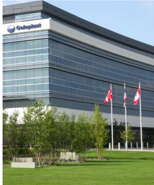
Medical technology firm Coloplast's new North American headquarters on a former brownfield site in Minneapolis. The 178,000 square foot building, containing office, R & D and production space, features river views and abundant natural lighting, and was designed to achieve Silver LEED certification. Assisted by city Tax Increment Financing and funding from the State of Minnesota and from Metropolitan Council. Photo by Metropolitan Council.
