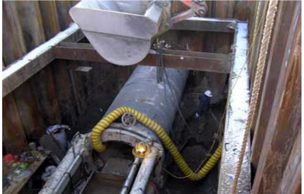
Heavy equipment pushes segments of the outfall pipe into the tunnel.
