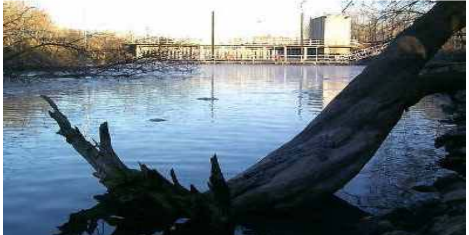
Photo of the Metro Plant effluent channel
