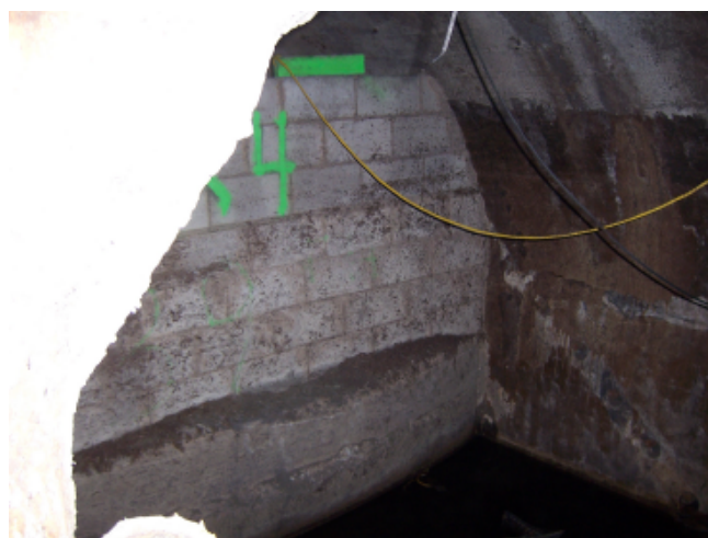
Figure 2.1-5. Regulator R04 Overflow Weir
