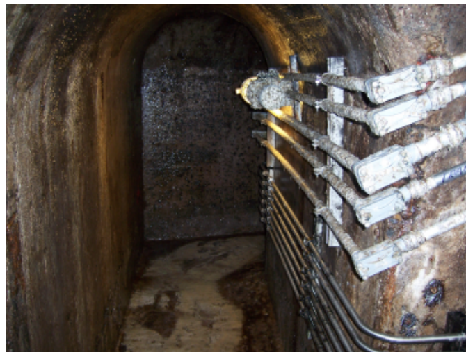
Figure 2.6-4. Additional odor control will reduce humidity and corrosion in the tunnels
