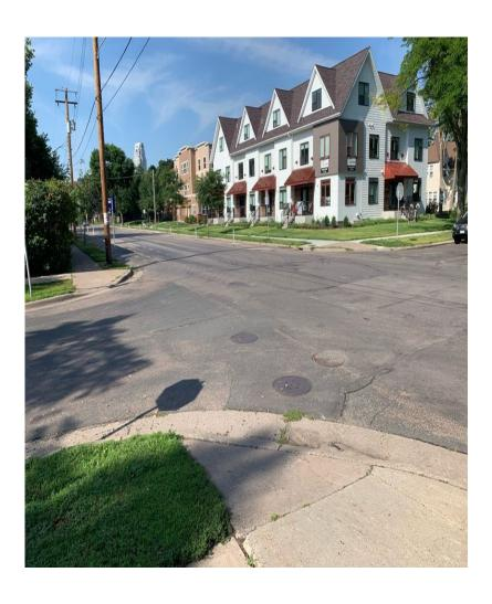
Photo of the intersection of 10th Ave SE and 7th St SE showing ADA non-compliant pedestrian ramps and a wide, difficult to cross street. 174 KB
